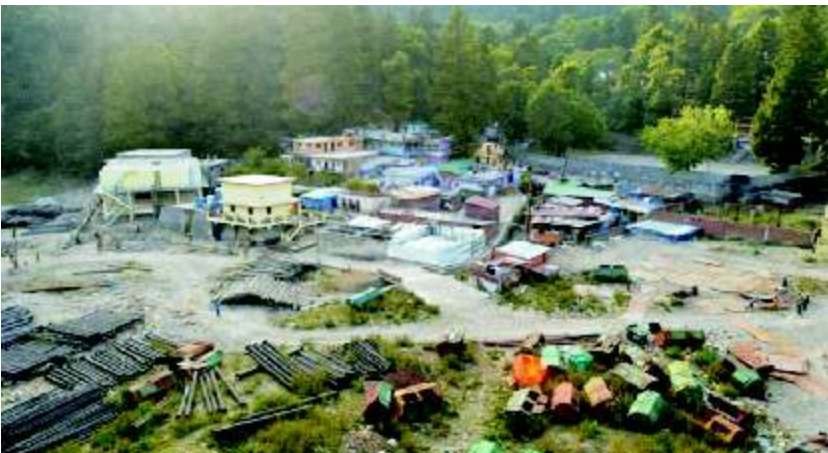
Figure 7. Construction activities in and around Sukhatal valley fill.
